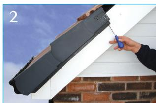
Clip together a second Dry Verge Unit and push it onto the tail of the first, until both sides of the clip engage with the tail fins of the first. Once again ensure the Verge Unit butts against the end of the tile. Then screw the tail end of the Verge Unit through the rear hole so it attaches to the barge board.
