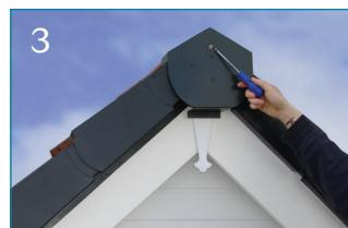
Repeat instruction 2 until all tiles have been covered. Once the Left Hand Verge is completed, repeat on the opposite Verge using the Right Hand Verge Units. The Ridge Cap is then securely screwed into the dry verge.
