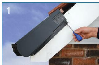
Apply starting piece and slide the Dry Verge Unit (pointing towards the apex) until the Verge Unit butts against the end of the first tile. Screw the Verge Unit through the top and bottom holes, so that the screw penetrates the barge board or brick and firmly holds the Dry Verge in place.
